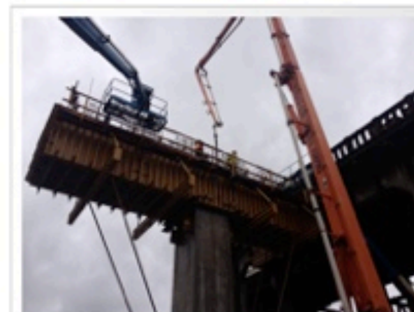
Pouring Bent 7 crossbeam for east approach
